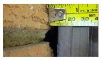
**Figure 9** A gap on the external wall surface between frame and brickwork.
