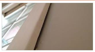
Figure 8 An internal gap between the architrave wall.
