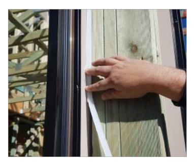
**Figure 12** Applying high density acoustic foam to the exterior of the window frame.
