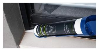
**Figure 10** Applying sealant to the external frame of a glazed sliding door.
