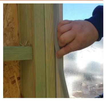
Figure 11 Applying high density acoustic foam
