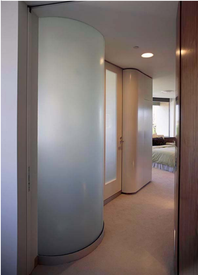
10mm clear toughened curved glass shower screen with applied frosted film Apartment Darling Point, NSW
