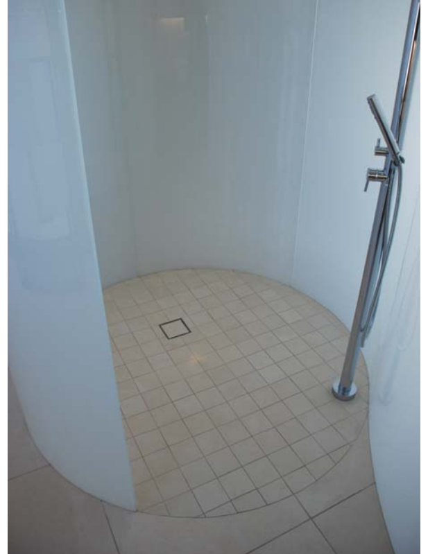
12.76mm starphire white translucent laminated curved glass inside view OEM Apartments, East Melbourne Vic
