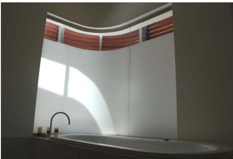
11mm clear laminated curved glass bathroom window with applied privacy film Private residence, Bronte NSW
