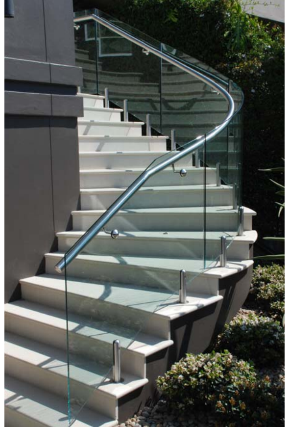
12mm clear toughened glass balustrade Private residence, Cremorne NSW
