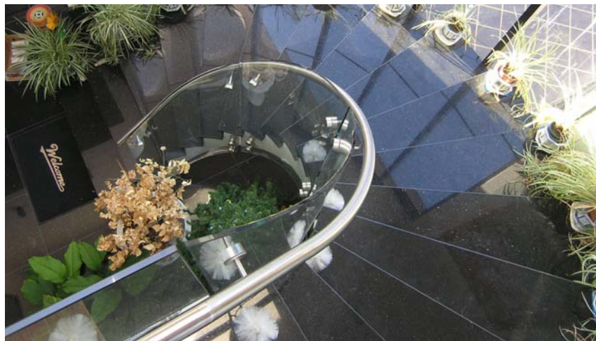
12mm clear toughened curved glass stair balustrade Private residence, Blakehurst NSW
