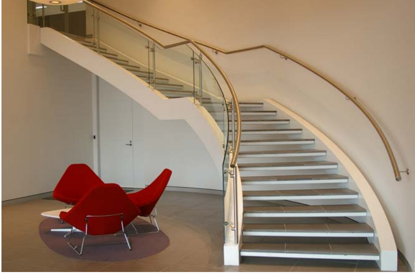
12mm clear toughened curved glass stair balustrade Office foyer, Gosford NSW
