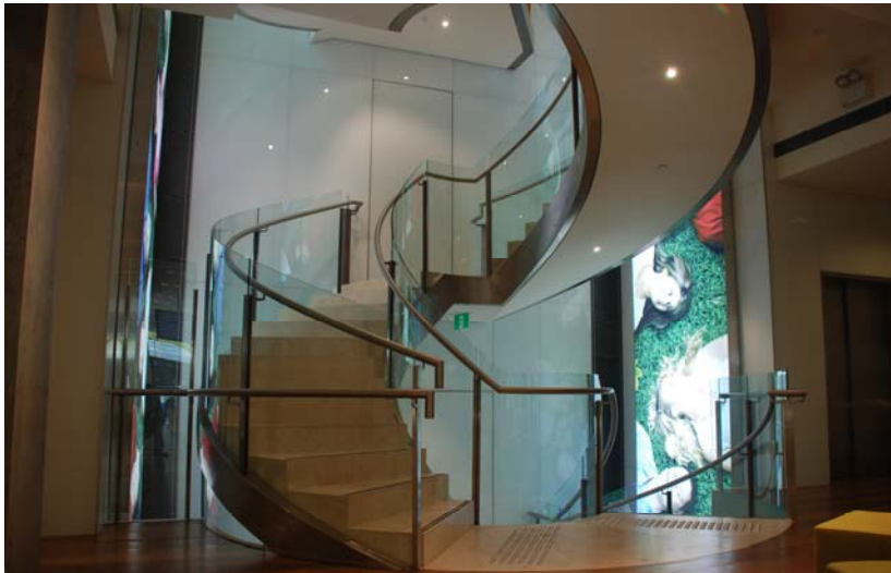
10mm clear toughened curved glass stair balustrade MBF Health Fund Headquarters, George St. Sydney NSW
