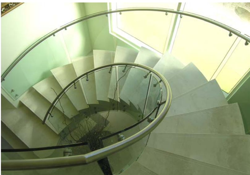
12mm clear toughened curved glass balustrade panels cantilever frameless panels Private residence, Sylvania Waters NSW
