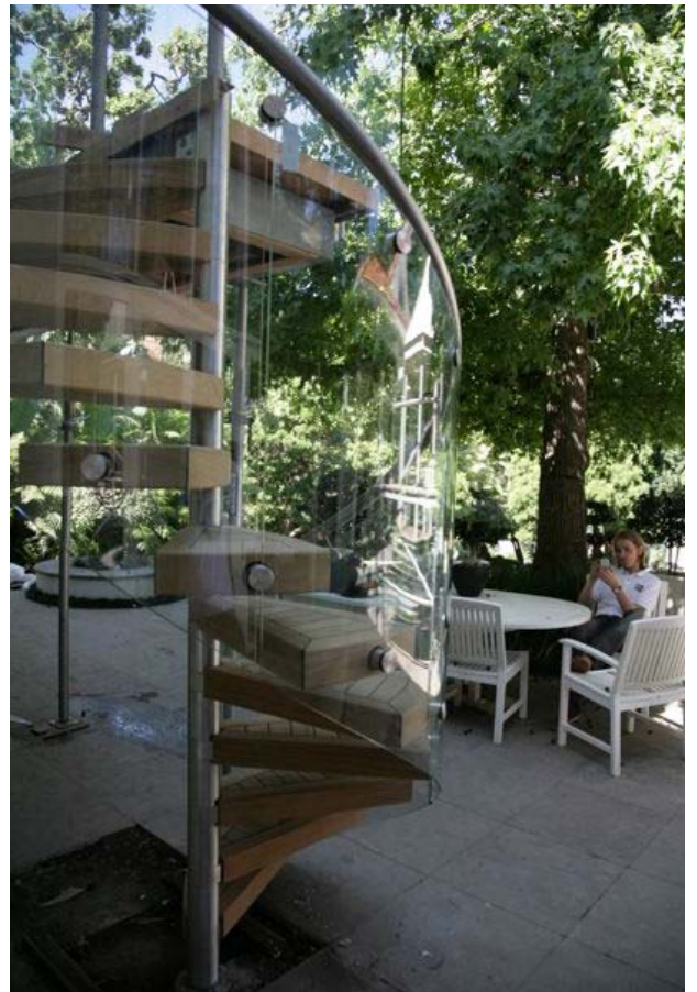
10mm clear toughened curved glass spiral balustrade Private residence, Wahroonga NSW
