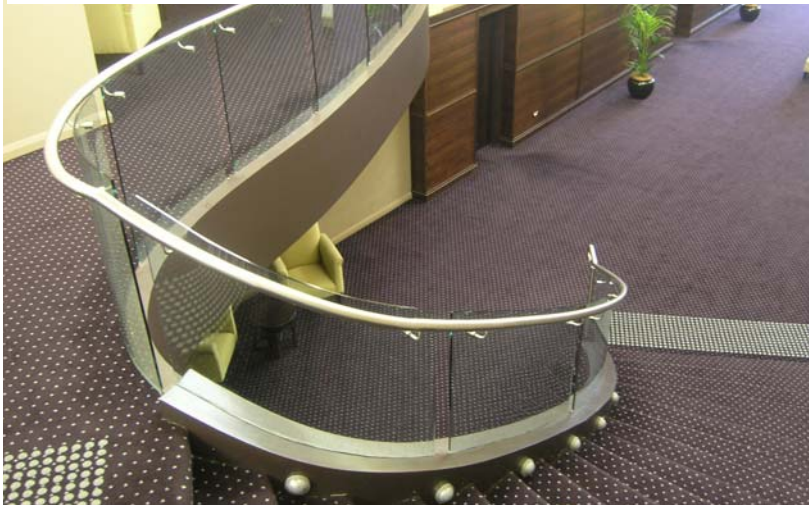
12mm clear toughened curved glass balustrade Miramare Centre, Terrey Hills NSW
