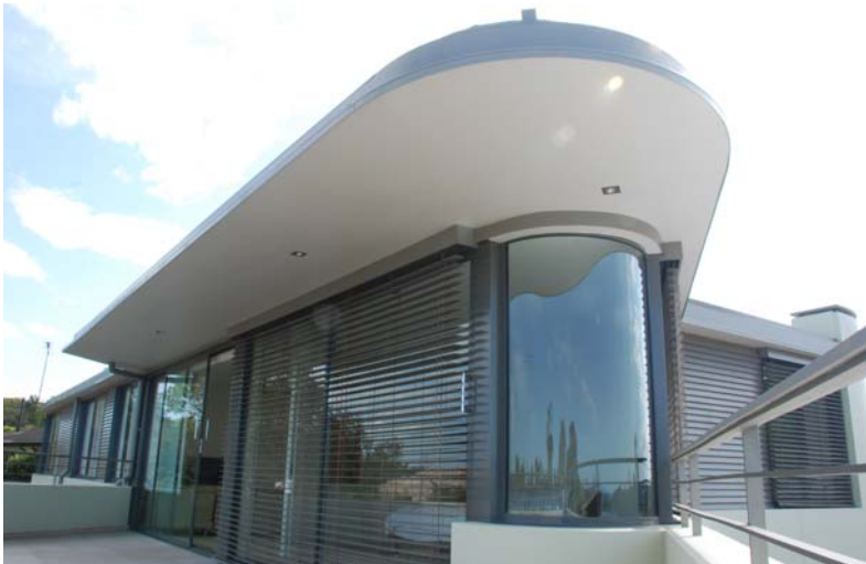
11mm clear laminated curved glass fixed panels silicon glazed into aluminium channel Private residence, Mosman NSW
