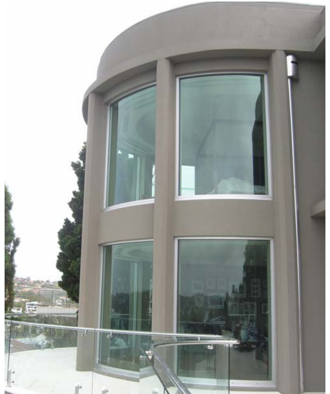
11mm Green tinted Low E laminated curved glass Private residence, Clontarf, NSW
