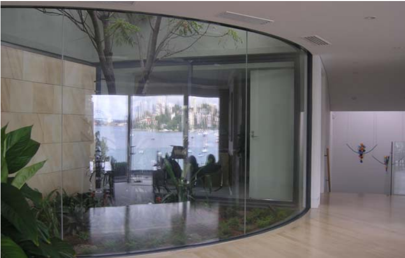
13mm clear laminated curved glass atrium Private residence, Sydney NSW
