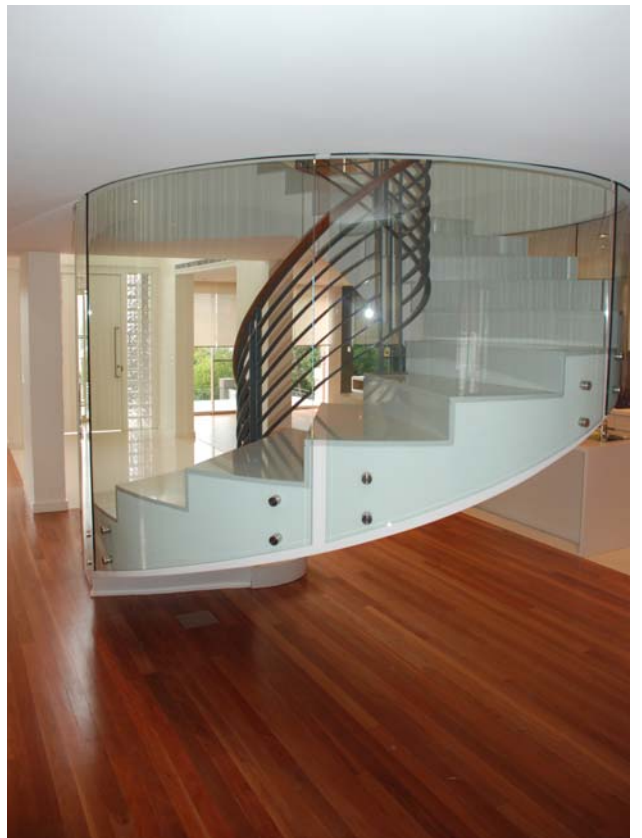
10mm clear toughened curved glass stair balustrade screen Private residence, Longueville NSW
