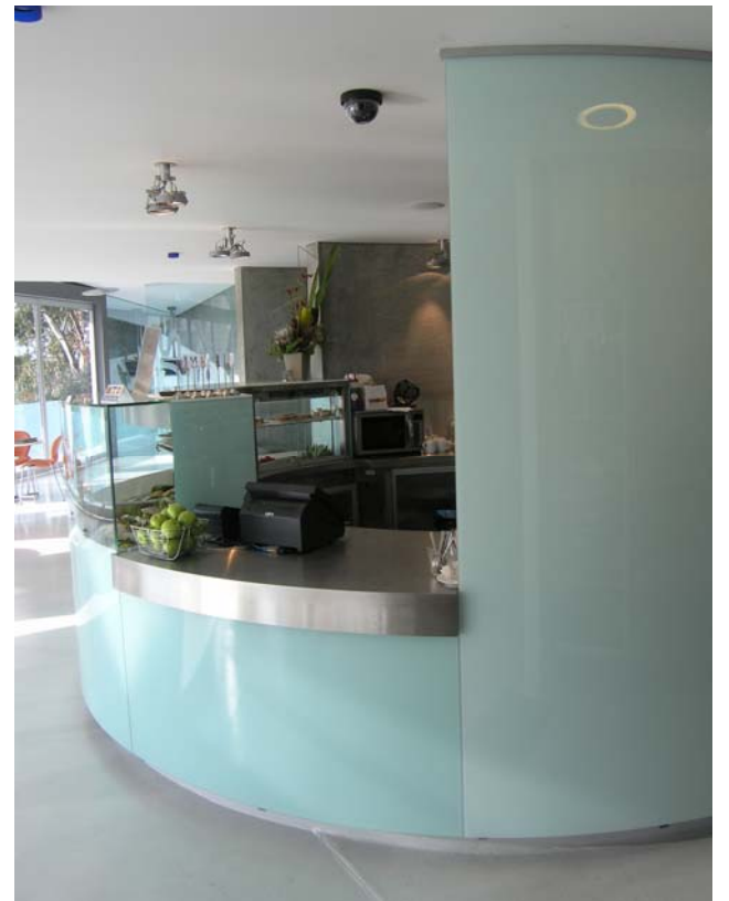
10mm clear toughened and colourback curved glass food counter Awash carwash & Café, Gladesville NSW
