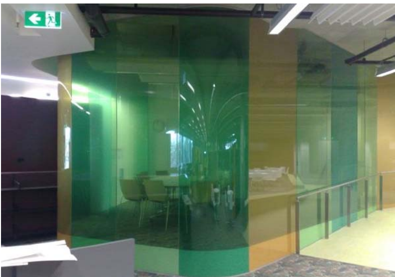
12.76mm laminated curved glass coloured interlayer Sydney University Library
