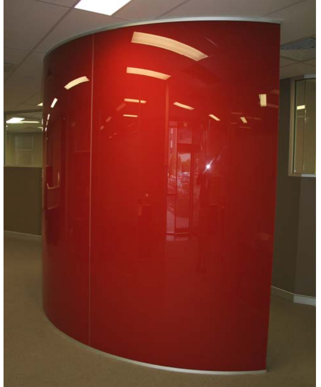
13mm opaque red laminated curved glass Safety Works Office, Newcastle NSW
