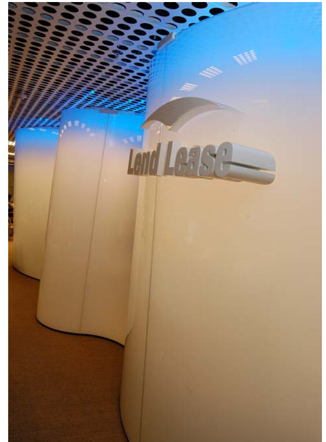
17mm curved laminated starphire glass panels with applied translucent film Lend Lease Head Office, Sydney
