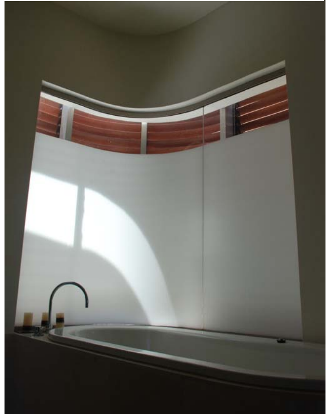
11mm clear laminated curved glass bathroom window with applied privacy film Private residence, Bronte NSW
