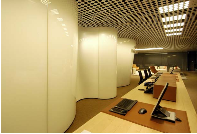
17mm curved laminated starphire glass panels with applied translucent film Lend Lease Head Office, Sydney NSW
