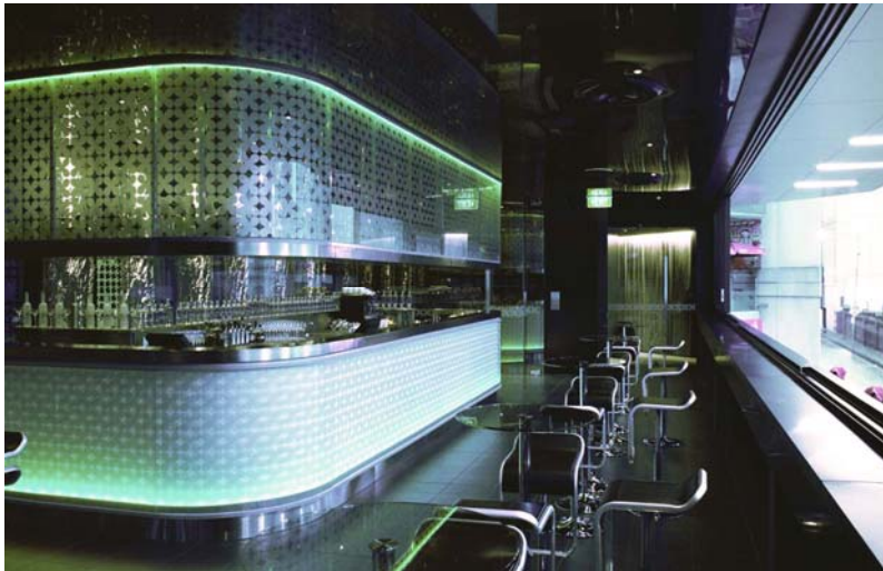
10mm clear toughened curved glass bar with applied decorative film Kaleido Bar, Melbourne Victoria
