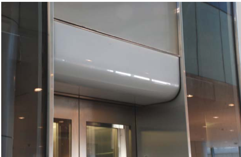
Alliance Centre No. 2 Market Building, Sydney NSW 6mm Starphire toughened curved glass frosted film to inner face, back illuminated
